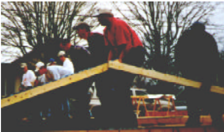
Staff from Division III help raise the roof of a house being built for Habitat for Humanity.
