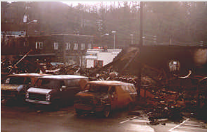
Community corrections officers in Mitchell County have a new home after a Christmas Eve fire destroyed their leased office space.
