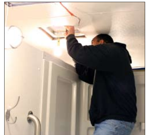
Above, an inmate installs a ventilation fan in one of the bath units. Below, volunteer Templeton Elliott, left, works with inmate Vann McDonald in preparing an electrical junction box for the laundry room in the shower trailer.
