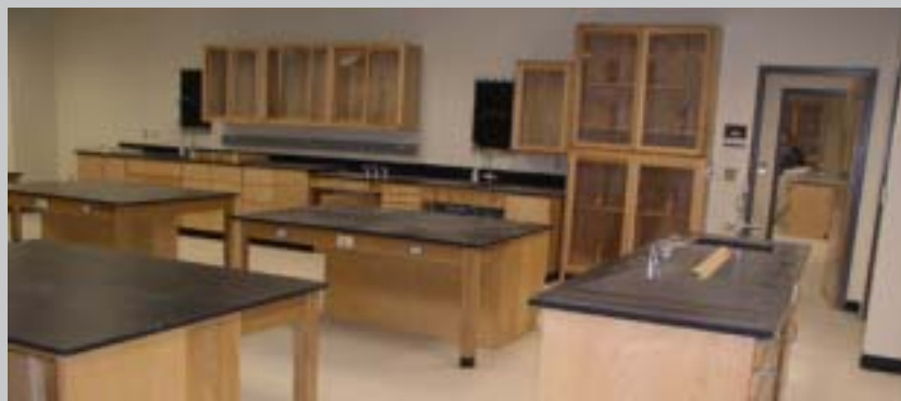
In a first of its kind contract, Correction Enterprises built and installed the lab tables, cabinetry and wooden casework for the new sciences building on the Winston-Salem State University campus.
