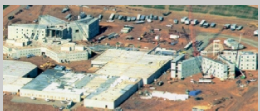
Alexander Correctional Institution is a 1,000 cell, close custody prison under construction in Taylorsville. Inmate occupancy is projected for Spring 2004. Similar prisons are also under construction in Scotland and Anson counties.
